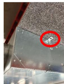
In normal operation the unit will not exhibit a significant level of vibration, however vibration mitigation treatment may be necessary in certain situations. Where units are installed with vibration limiting equipment, flexible connections should be applied to all other services connected.
