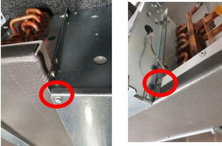
To remove the drain tray you first have to remove the fan access panel as previously described.
