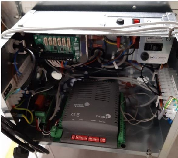
Check for blown fuses. If a fuse is blown check the circuits and components it protects thoroughly before re energising. Any blown fuse must be replaced with an equivalent fuse of the same specification, size and rating.
