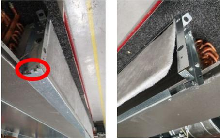
The filter is removed by undoing the two retaining screws situated beneath the filter that allows a hinged section to be pulled down giving access to the filter.
